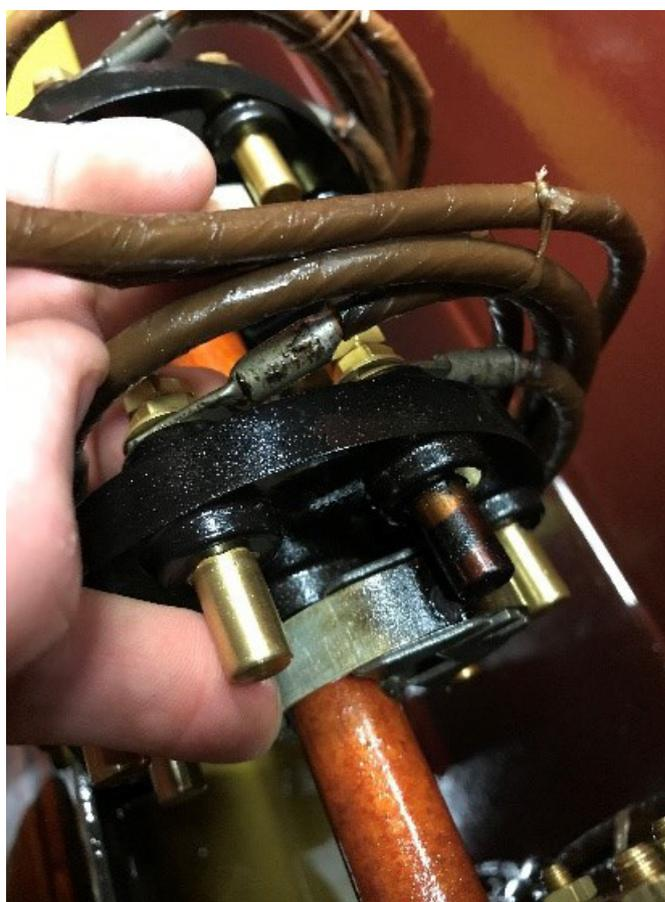
*Image: Off load tap changer where fault was located*
