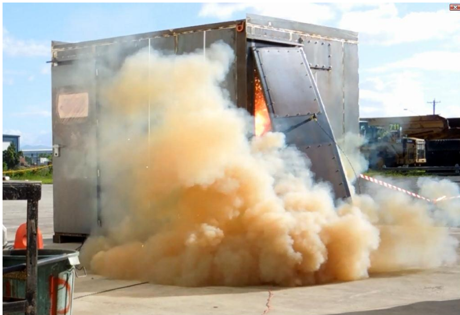
Figure 5: Unvented switchroom with simulated 22kA fault.
